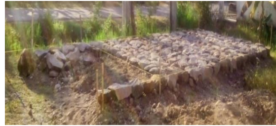
Fig.1. Base of the dryer room
