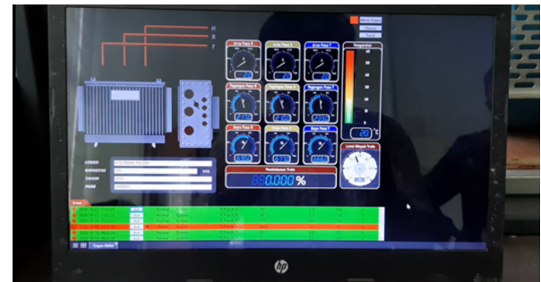
Fig. 7. Data shown in SCADA.
